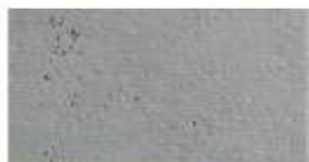
Coarse concrete technique
